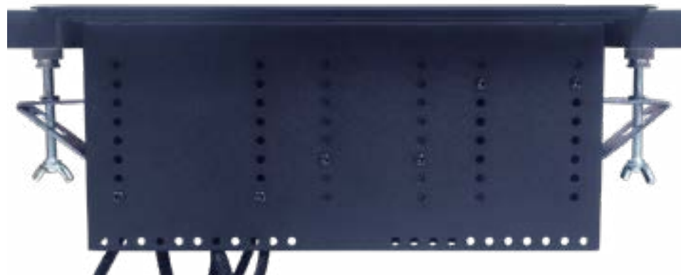
Brackets tightened & installed
